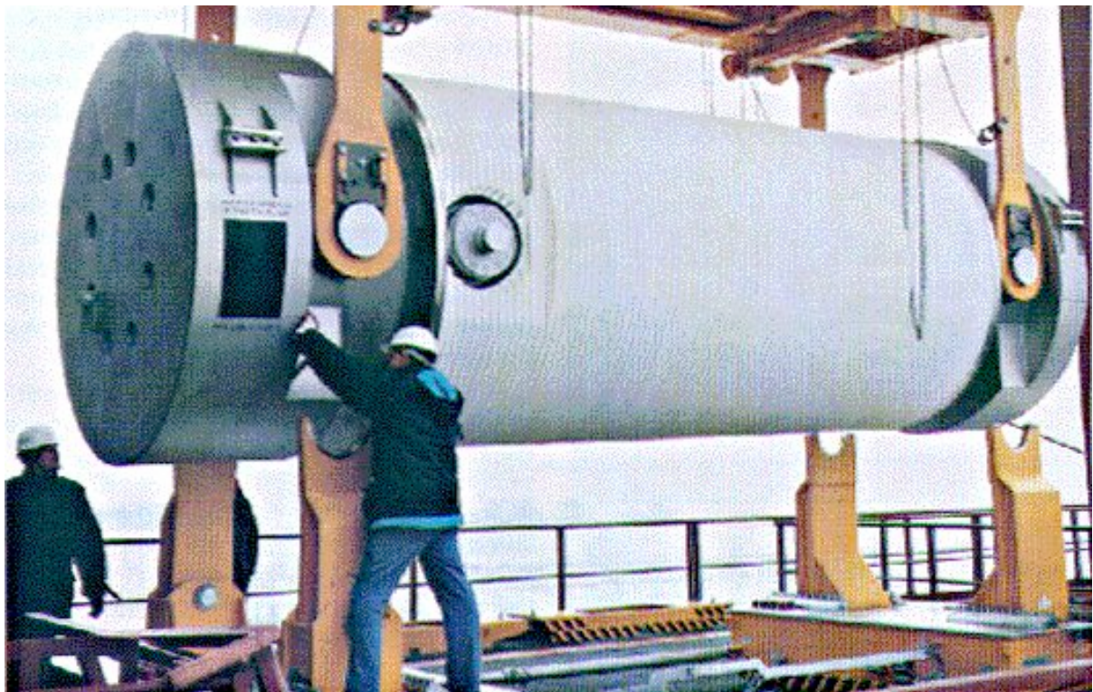
Figure 5.4: HLW transport container during shipping
